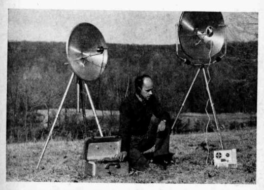
Elaborate echo-study equipment is shown above operated by the author. On the right, a radar with speaker is used to beam sounds
